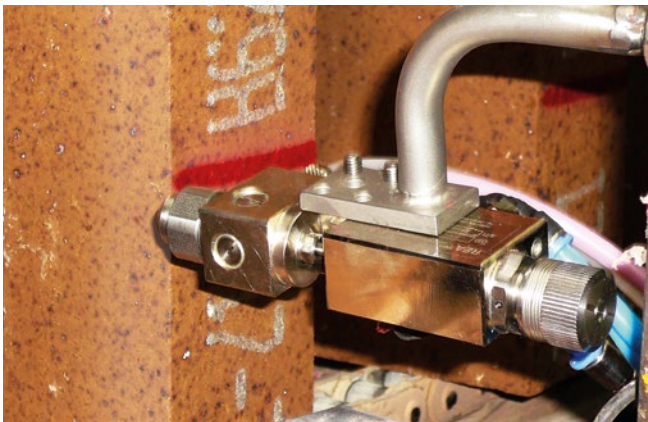
Chimney stone line-marking for correct installation
